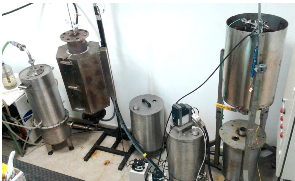
Figure 3.1. Glycerol steam reforming pilot plant.
